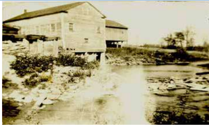
A flood washed out the dam in 1912.
