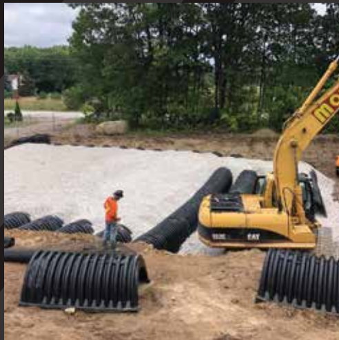
Septic Design & Installation
